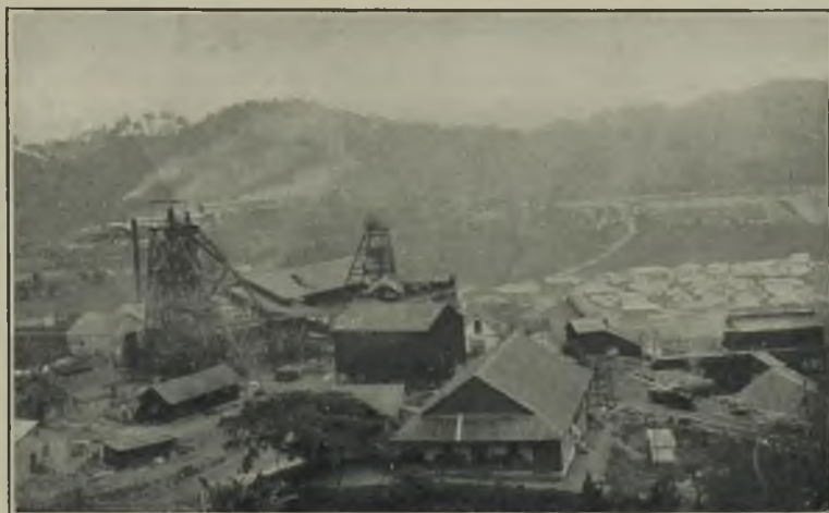
GENERAL VIEW OF THE ASHANTI MINE AND SURFACE BUILDINGS.
