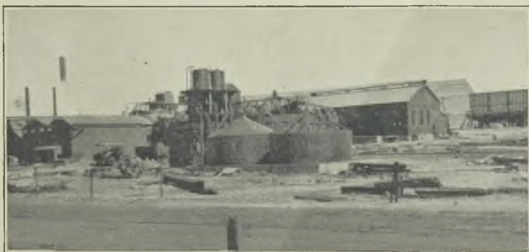
FIG. 10.—POWER PLANT, WITH MILL OIL TANKS IN FOREGROUND.
