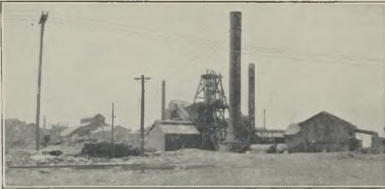
FIG. 8.—CHAFFERS BOILER PLANT AND OLD HEADFRAME.
