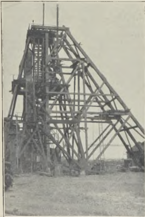
FIG. 2.—ERECTION OF CHAFFERS HEADFRAME.
