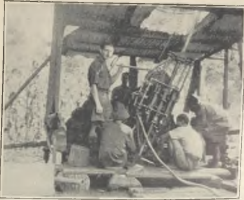
FIG. 2.—DRILLING AN INCLINED HOLE.
