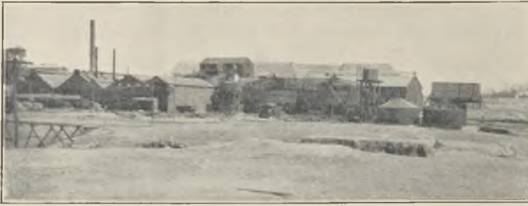
FIG. 1.—POWER PLANT AND MILL, WITH BOULDER TAILINGS DUMP IN BACKGROUND.
