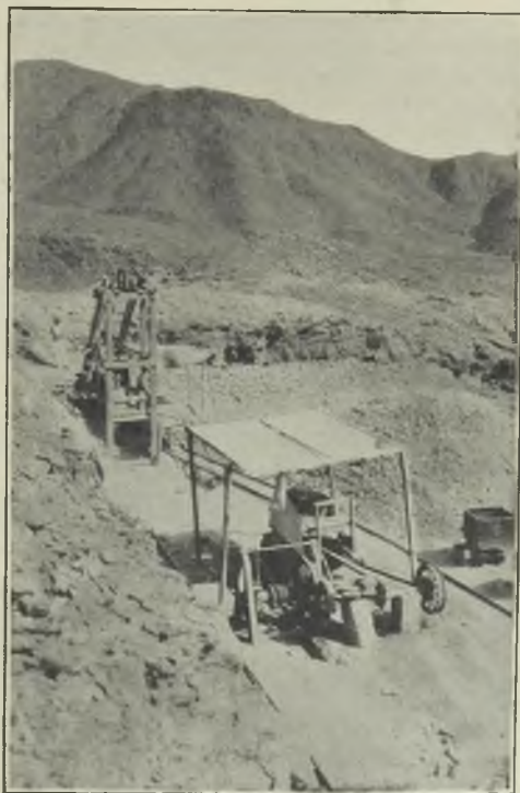
FIG. 9.—MAIN SHAFT HOIST AND HEADFRAME AT WADI OYO. THE HOIST IS A MODEL T FORD MOUNTED ON CONCRETE BLOCKS.
