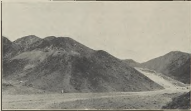
FIG. 7.—WADI OYO MINE. ANCIENT WORKINGS ARE SHOWN ON THE LEFT AND ON THE RIGHT THE MODERN WORK BEING DONE BELOW THEM.
