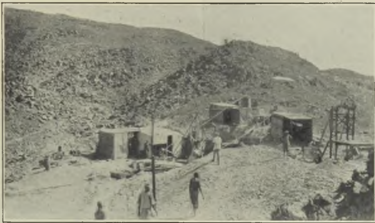
FIG. 2.—MILL AND HEADFRAME AT THE GARABIEN MINE.
