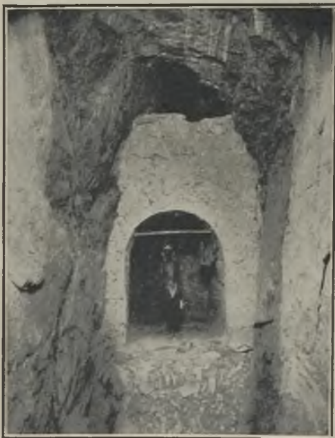
FIG. 9.—74TH LEVEL, SOUTH SECTION, SHOWING CONCRETE ARCHING.
