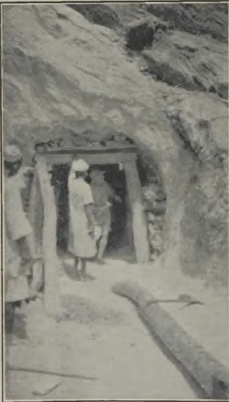
FIG. 4.—ADIT IN TALC-CARBONATE ROCK.
