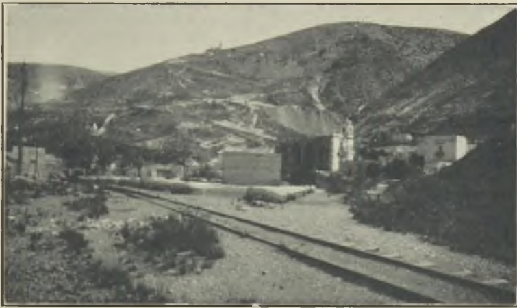
EASTERN SECTION OF CATORCE AT END OF GREAT TUNNEL.
