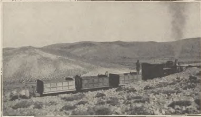
FIG. 3.—LIGHT RAILWAY TRANSPORT.
