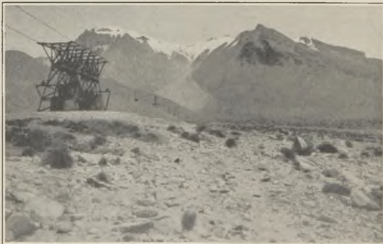
FIG. 4.—AERIAL ROPEWAY FROM THE MINES.
