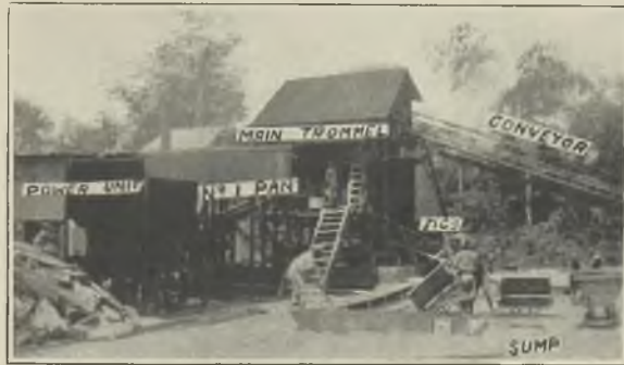
FIG. 1.—DETAILS OF A PAN PLANT.
