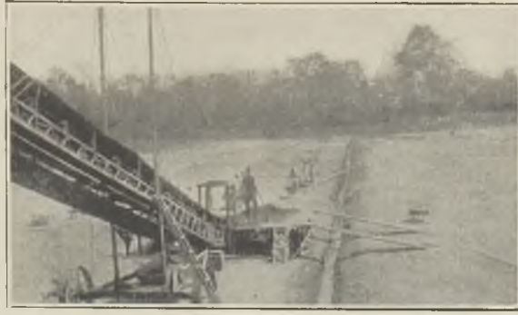
FIG. 9.—PAN PLANT: ELEVATION OF GRAVEL BY BELT-CONVEYOR.
