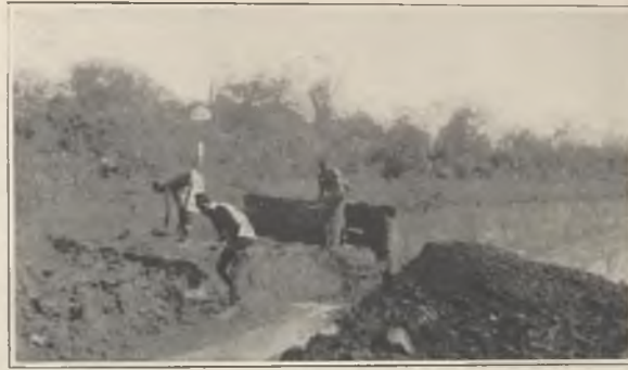
FIG. 15.—EXCAVATING OVERBURDEN UNDER CONTRACT.
