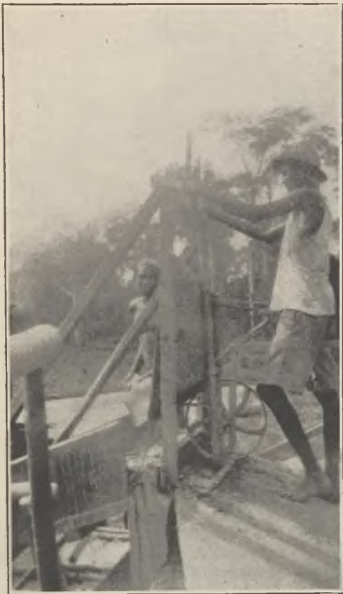
FIG. 11.—UNLOADING GRAVEL INTO PUDDLE-BOX.
