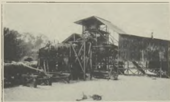
FIG. 4.—PAN PLANT WITH TWO WASHERS IN SERIES.
