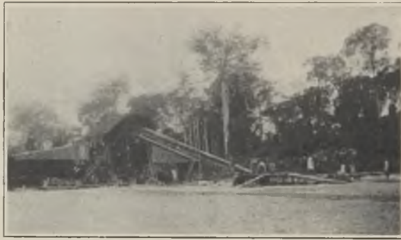
FIG. 5.—PAN PLANT, SHOWING LOADING PLATFORM AND CONVEYOR.
