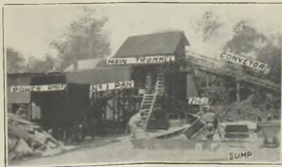
FIG. 1.—DETAILS OF A PAN PLANT.
