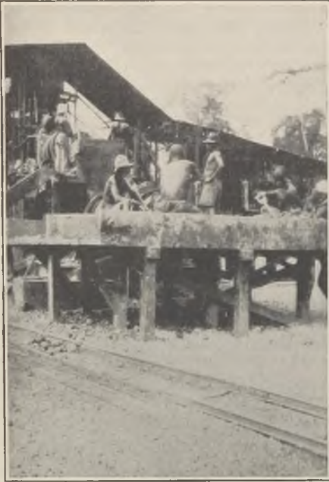
FIG. 2.—HAND-PICKING DISCHARGE FROM SECOND WASHER.
