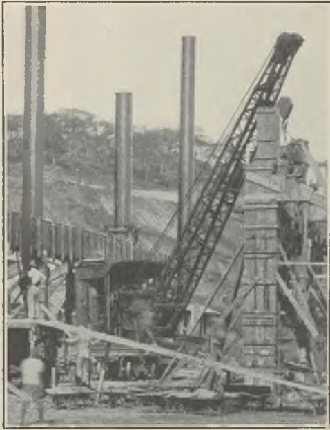
FIG. 6.—EXCAVATOR FITTED AS CRANE ON A CONGO MINE.
