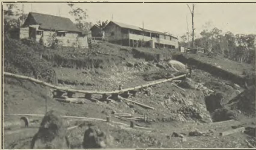
FIG. 8.—SLUICING OVERBURDEN AT GOLDEN RIDGES.
