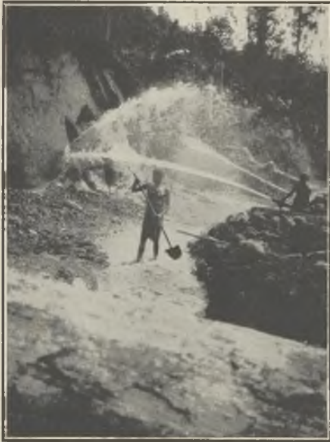
FIG. 11.—MONITOR WORKING ON THE BULOLO.
