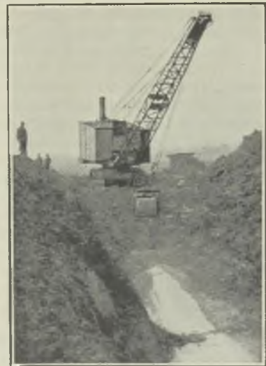
FIG. 5.—MENCK AND HAMBROCK DRAGLINE DIGGING A CANAL.
