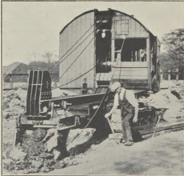
FIG. 3.—RUSTON-BUCYRUS EXCAVATOR FITTED AS A SKIMMER-SCOOP.
