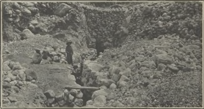
FIG. 7.—WASHING CHANNEL FROM A BURMESE WORKING OF THE "HMYAWDWIN" TYPE, YEGYI, NEAR MOGOK.
