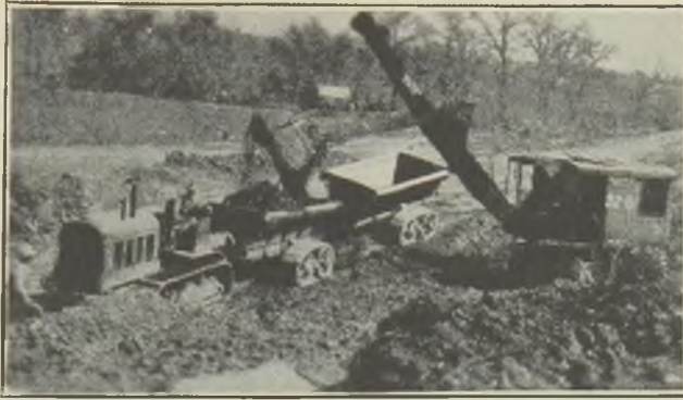
FIG. 11.—CRAWLER WAGONS FOR HAULING EXCAVATED GROUND.
