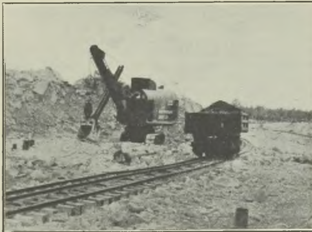
FIG. 12.—ELECTRICALLY-EQUIPPED WAGON OPERATED FROM CONTROL TOWER.
