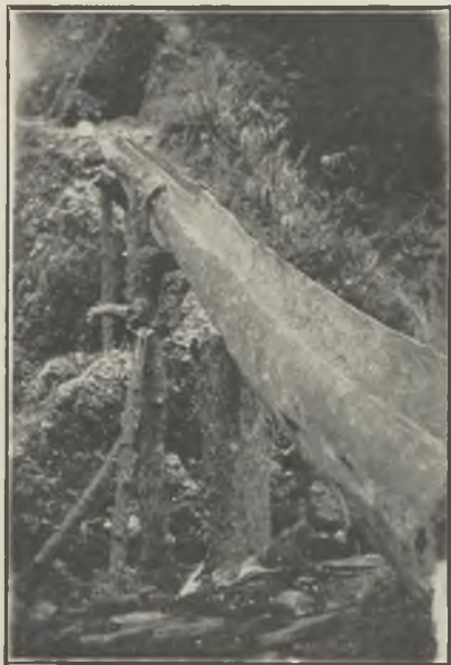
NATIVE FLUME FOR HYDRAULIC OPERATIONS.
