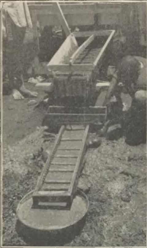
FIG. 4.—ROCKER WITH STATIONARY TESTING SLUICE, KAKAMEGA.
