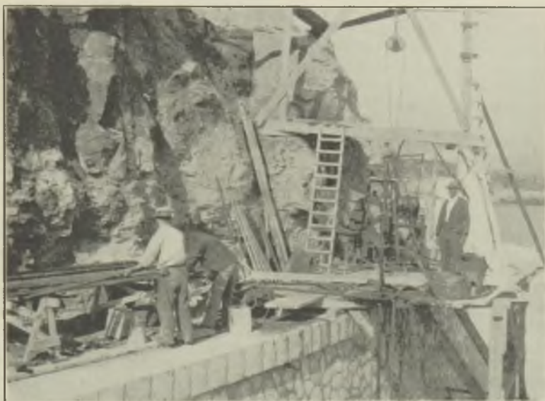
FIG. 2.—DRILLING A HOLE ON THE SPILLWAY RETAINING WALL.
