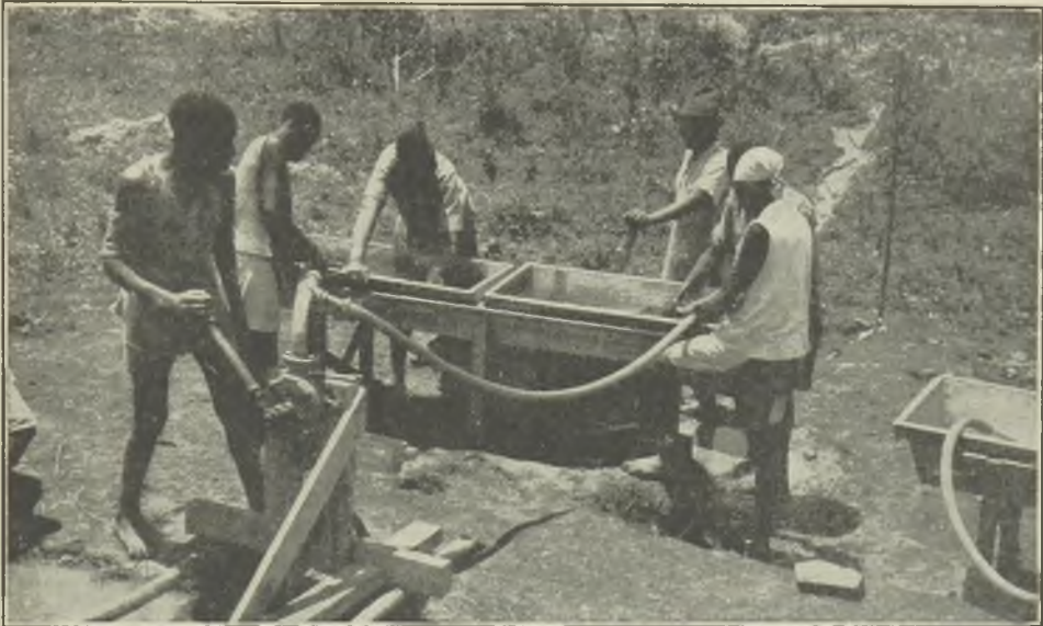
FIG. 7.—PUMP FEEDING ROCKER, KAKAMEGA.
