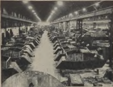
The fabrication and welding 'line-up' at Birtley.
