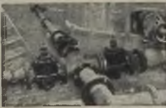
6" 'Audco' Valves on Salt Liquors.
