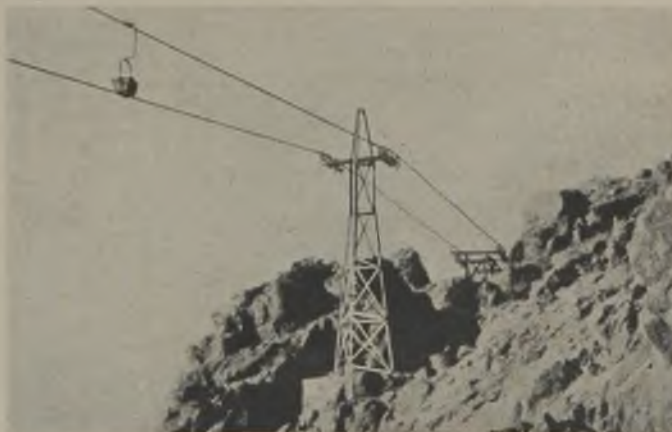
VIEW OF MONOCABLE ROPEWAY IN BOLIVIA LENGTH—8,000 metres
