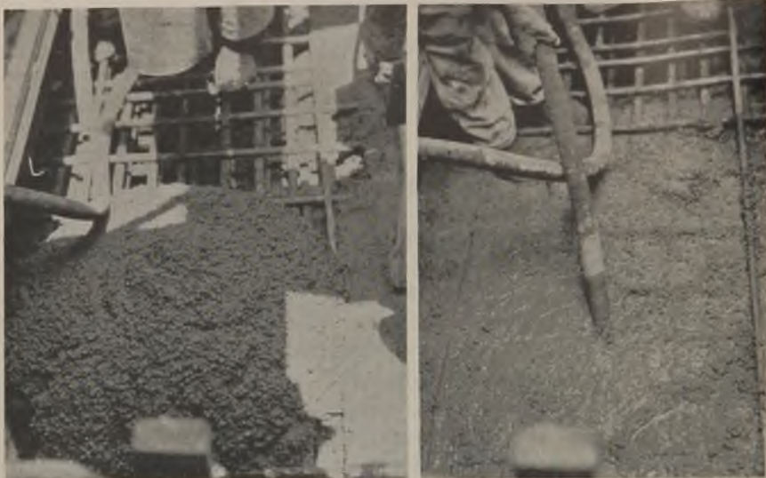
Fig. 22 (left)—Newly deposited concrete in bottom flat, Tampa (step 2, Fig. 21). Note medium-low-slump, small-maximum-size, nodulite concrete.
