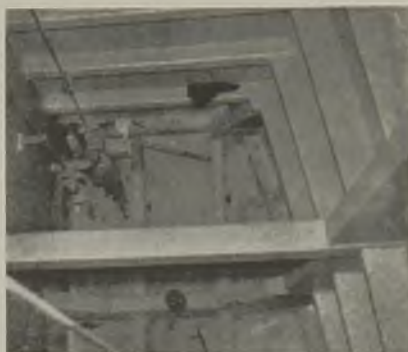
Fig. 39 (left)—Vinylite resin paint (black) was used on interior of cargo tanks in the National City oil barges.
