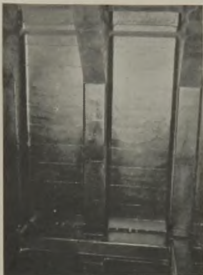
Fig. 39 (left)—Vinylite resin paint (black) was used on interior of cargo tanks in the National City oil barges.
