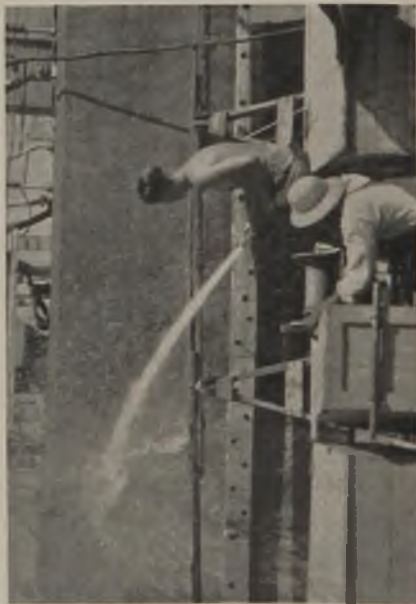
Fig. 28 (top left)—Water curing of hull interiors commenced as soon as forms were stripped. Structural details of interior National City oil barge are shown.
