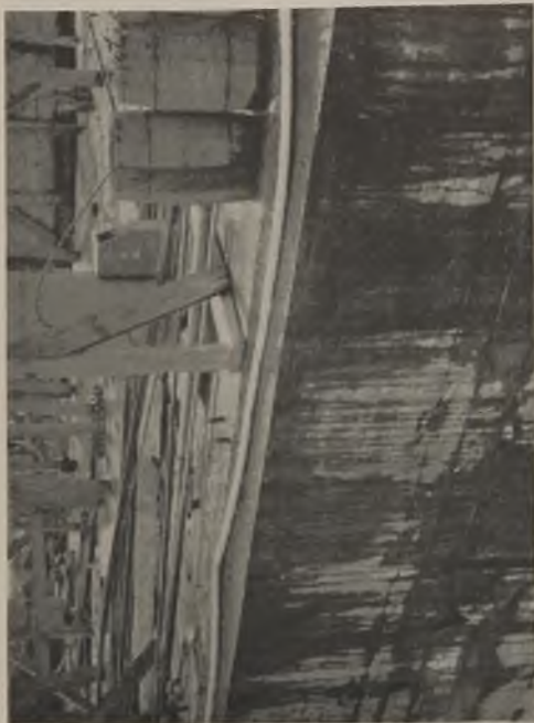
Fig. 28 (top left)—Water curing of hull interiors commenced as soon as forms were stripped. Structural details of interior National City oil barge are shown.
