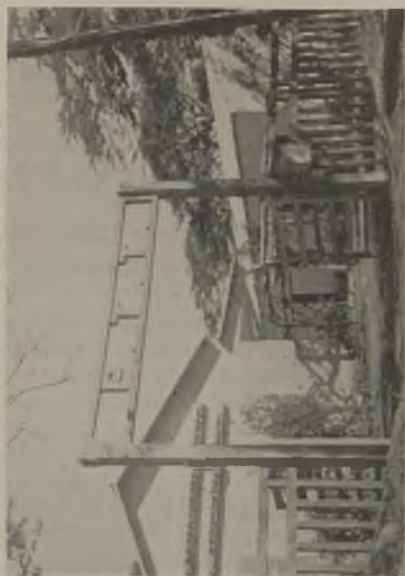
Fig. 3—Post-office gate, sign, fence and the post-office itself in La Foa are all of concrete.
