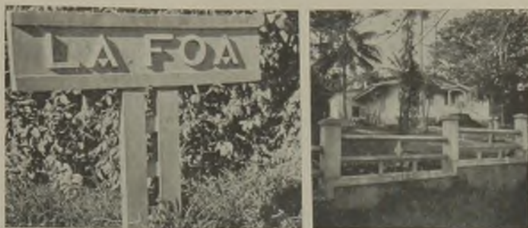
Fig. 5—Signpost on the outskirts of La Foa, a village of perhaps 250 people, 80 miles north of Noumea, is cast in one piece of solid concrete, and stands as high as a man's shoulders. The supports and background for the matrix letters are natural concrete; the letters are painted a light blue and the two horizontal bars dark blue.
