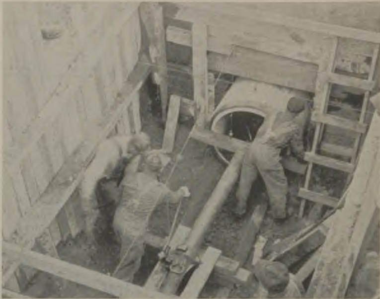
Fig. 1—Jacking 36-in. diameter precast concrete pipe under railroad tracks
