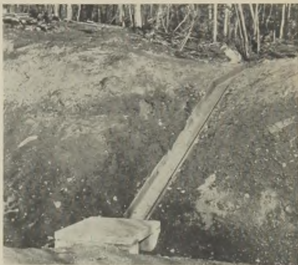
Fig. 3—Culvert Intake and drain on Forest Highway, New Hampshire.
