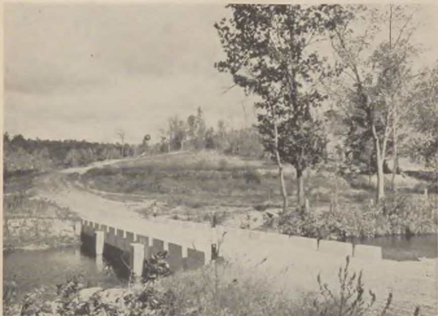
Fig. 1—Smallwood bridge on Spring Creek, Missouri. It is typical of the low water bridges used where the floodwaters cover so much of the wide valleys that high water bridges would be extremely long and their high cost could not be justified by the traffic. Gage posts on each end of the bridge indicate the depth of the water over the bridge in the early stages of the flood and serve as a guide to the motorist as to his chance of crossing the river.
