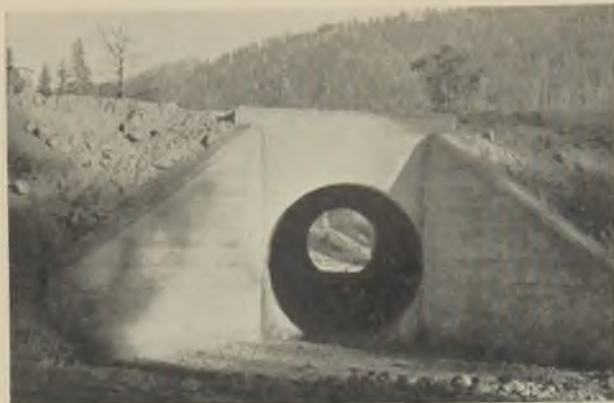
Fig. 3—Culvert Intake and drain on Forest Highway, New Hampshire.
