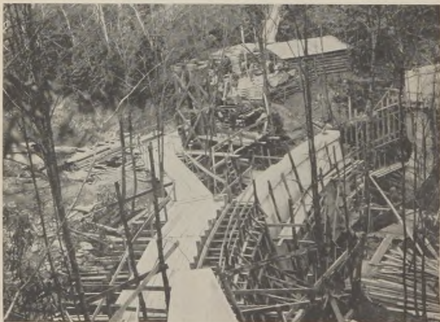
Fig. 5—High Knob Dam, Jefferson Nat'l. Forest, Virginia. Aggregates delivered down hillside by chute to mixer platform; cement stored in log cabin; concrete wheeled to forms; skip serves various levels.
