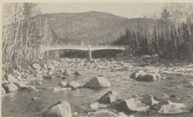
Fig. 11—Two (90-ft.) span rigid frame concrete bridge constructed by Forest Service over E. Branch Pemigewasset River, Swift River Forest Highway, near Lincoln, N. H. White Mtn. Nat'l Forest.
