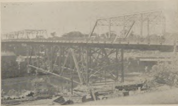
Fig. 1—General view of Spruce Street Bridge
