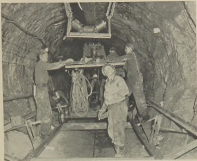
Fig. 9—9-inch steel paving forms used for the west end of tunnel invert lining.
