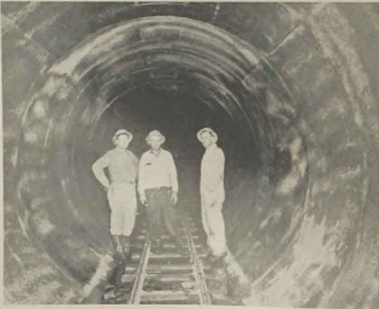
Fig. 19—The completed lining is relatively free from imperfections and a glossy finished surface is produced by the form oil.
