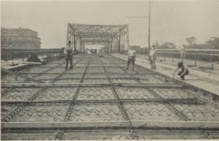
Fig. 3—Looking north across the deck span
