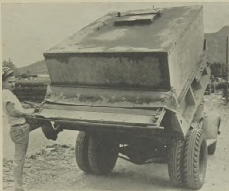
Fig. 4—Cement was transported in standard dump trucks fitted with a specially constructed water tight cover.
