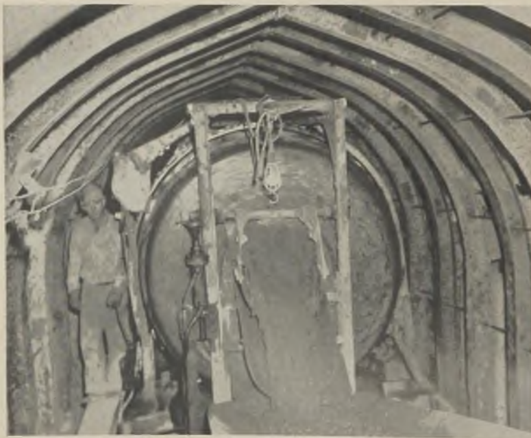
Fig. 12 (top)—A Rex mixer was used on the west end of the work. Water batching tanks were lowered to provide clearance between mixer and tunnel roof.
