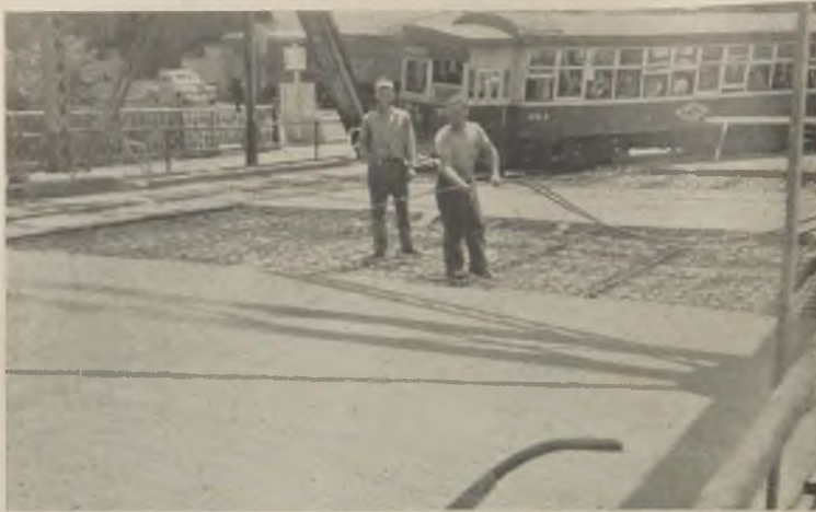
Fig. 10—Curing by oil spray
