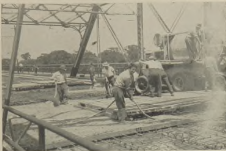
Fig. 8—Placing concrete slab
