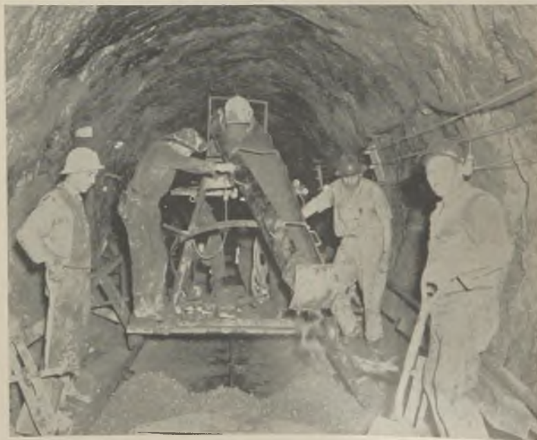
Fig. 14 (top)—Placement of invert lining on the east end.
