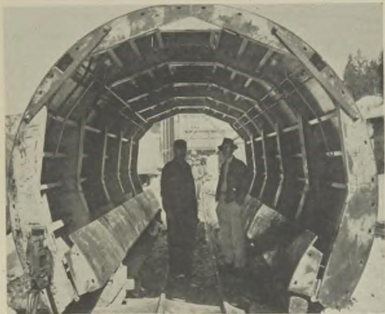
Fig. 10—An assembled arch and sidewall form.
