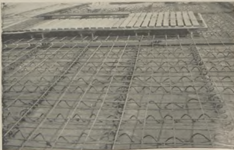
Fig. 7—Slab section ready for concreting
