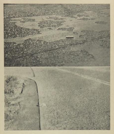
Fig. 4 (top) – Type 3 deterioration. Partial removal of mortar top from pavement due to excessive use of chloride salts for ice removal. Pavement built in 1934, photographed in 1944.
