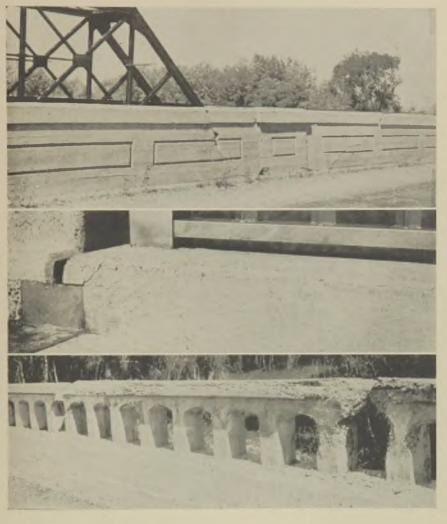
Fig. 1. (top) – Type 1 deterioration. Structural damage due to colliding vehicle. Concrete sound. Bridge built in 1921, photographed in 1944.
