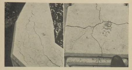
Fig. 6. (left)—Type 4 deterioration. Wide, open cracks in wing wall. Concrete otherwise sound.
