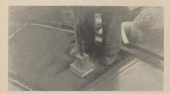
Fig. 5—Test specimen 4 using Ecement. Mix by weight 1:2.7, maximum size of aggregate 14 in., w/c ratio 0.30, moist earth consistency. This photograph shows how the topping was tamped.
