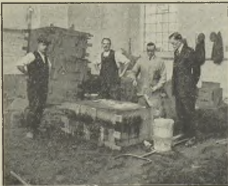
FIG. 4.—POURING A TEST-BAR IN A CHILL-MOULD.
