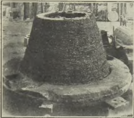
FIG. 2.--THE CORE REMOVED FIVE HOURS AFTER CASTING.
