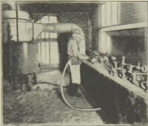
FIG. 16.—SAND-BLAST ROOM WITH WORK BENCH FOR SMALL CASTINGS AND DUST COLLECTING ARRANGEMENT.
