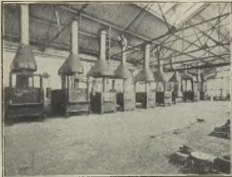
FIG. 11.—VIEW OF A BATTERY OF CARBURISING AND NORMALISING FURNACES.
