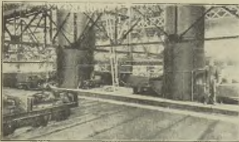
FIG. 17.—AMERICAN METHOD OF HANDLING CUPOLA TRUCKS.
