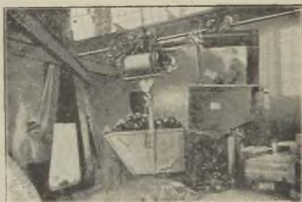
FIG. 19.—ELECTRIC OVERHEAD RUNWAY.
