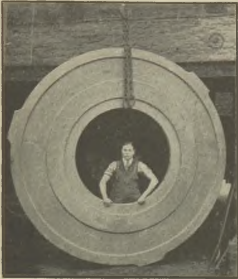
FIG. 9.—ALTERNATOR END RING IN NON-MAGNETIC CAST IRON. IT WEIGHS 3 TONS 12 CWT.
