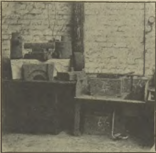
FIG. 8.—CORES AND A CORE JOLTING MACHINE.
