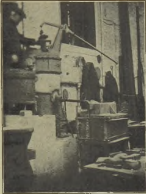
FIG. 17.—FILLING A BEARING.
