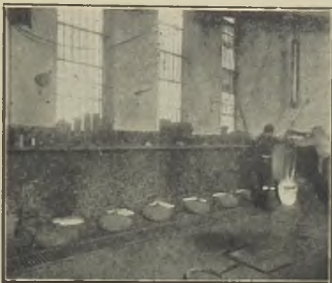
FIG. 3.—CRUCIBLE MELTING PLANT AT THE NORTH BRITISH LOCOMOTIVE COMPANY, LIMITED, GLASGOW.
