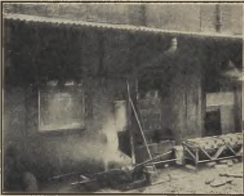
FIG. 4.—PART OF THE REVERBERATORY FURNACE PLANT AT THE NORTH BRITISH LOCOMOTIVE COMPANY, LIMITED, GLASGOW.
