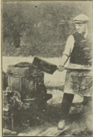
FIG. 16.—ANNEALING PAN MAKING. FILLING IN THE MOULD.
