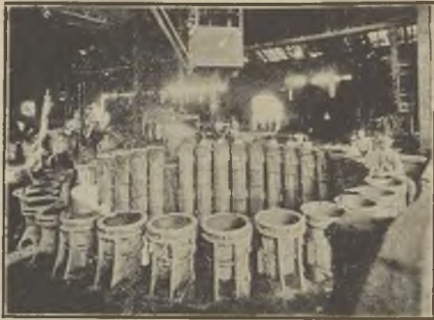
FIG. 6.—SAND CAST PIPE PIT.
