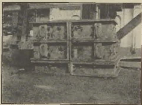
FIG. 13.—PARTIAL ASSEMBLY OF THE MOULD.
