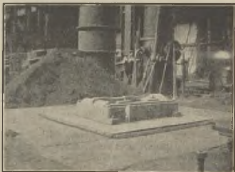
FIG. 6.—A PATTERN MOUNTED ON THE PLATE READY FOR RECEIVING THE BOX.
