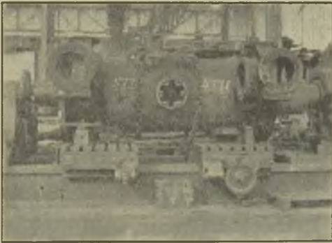
FIG. 11.—SHOWING CYLINDER CASTING.
