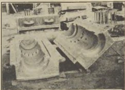
FIG. 9.—LINER MOULD.
