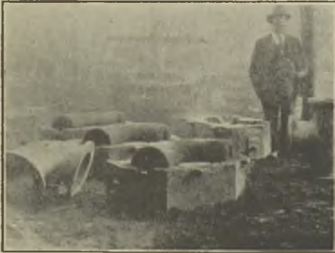
FIG. 10.—MOULDS FOR 12-IN. ELBOW CORES.
