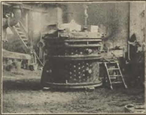
FIG. 12.—THE ASSEMBLED CORE READY FOR CASTING.
