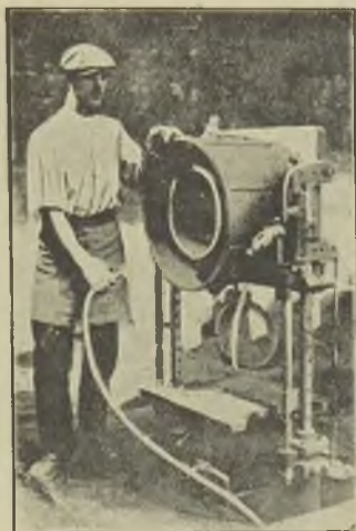
FIG. 20.—ANNEALING PAN MAKING. MACHINE TABLE TILTED.
