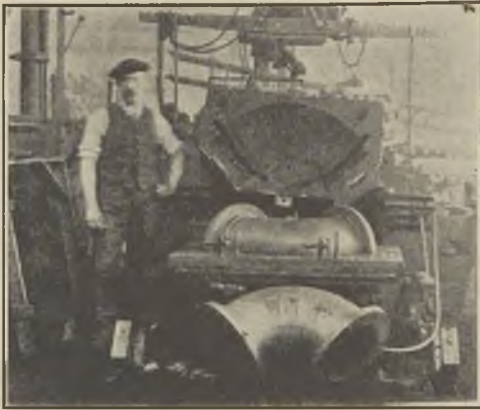
FIG. 9.—MAKING A 12-IN. ELBOW CORE.
