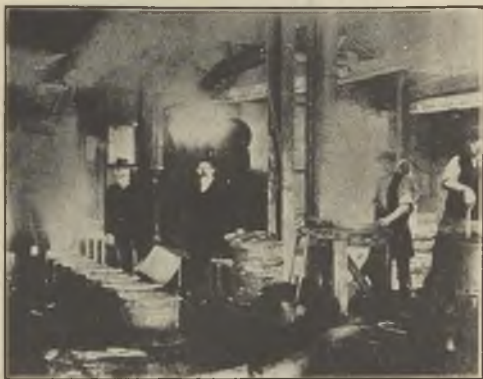
FIG. 21.—ANNEALING PAN MAKING. POURING THE MOULDS.
