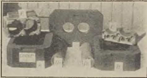
FIG. 1.—TOP MIDDLE PART; BOTTOM MIDDLE PART AND TOP CAKE CORE.
