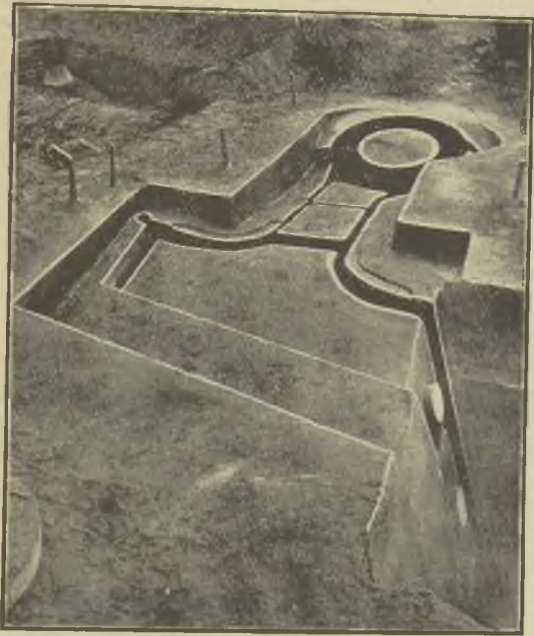
FIG. 2.—MOULD READY FOR CLOSING.
