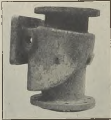
FIG. 6.—CLACK-TYPE RETENTION VALVE.
