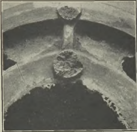
FIG. 11.—THE CONNECTING RIB BETWEEN TWO HEAVY SECTIONS IS TORN.
