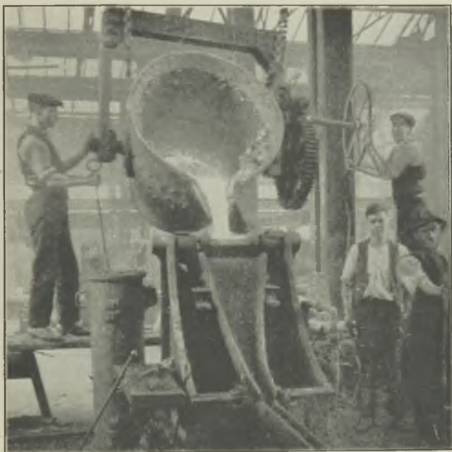
FIG. 17.—FALL SPOUT, AND FILLING OF TILTING HOPPER.
