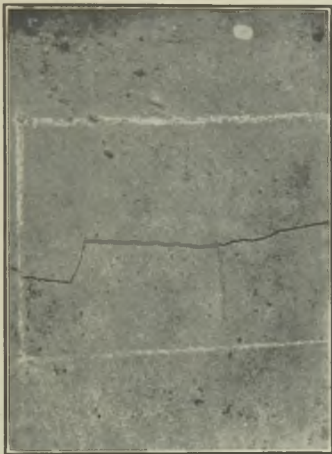
FIG. 15.—CONTRACTION STRESS CRACK.
