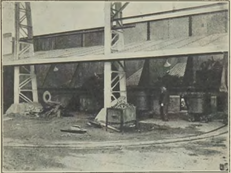
FIG. 2.—SHOWS THE SLOPING BINS AND SPECIAL CONTAINERS TO HANDLE RAW MATERIALS.
