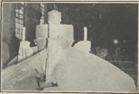
FIG. 13.—A 15-FT. DIA. FOUR-BLADED PROPELLER AFTER REMOVAL FROM THE PIT.
