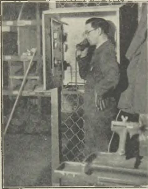
FIG. 4.—A TELEPHONE BOOTH IN THE FACTORY FOR COMMUNICATING WITH THE TIME BOOKING CENTRE.
