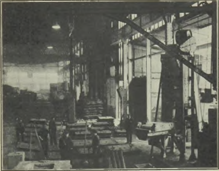
FIG. 18.—SHOWS A VIEW OF THE MAIN BAY OF THE FOUNDRY.
