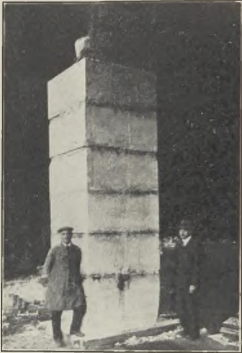
FIG. 4.—LARGE ROLL CASTING MOULD AFTER BEING CAST.
