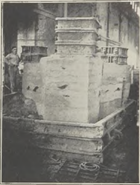
FIG. 24.—STERN TUBE BRACKET IN CAST STEEL, PARTIALLY STRIPPED.
