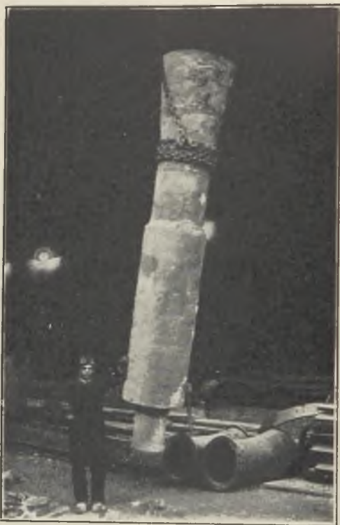
FIG. 6.—CASTING STRIPPED FROM MOULD.
