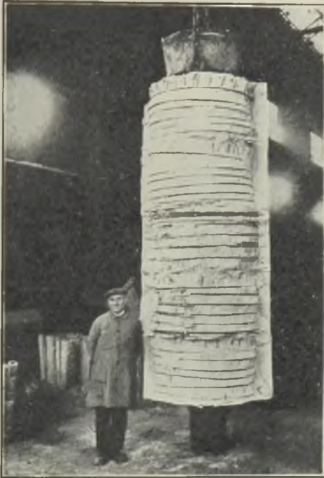
FIG. 5.—SAME MOULD AS SHOWN IN FIG. 4 PARTLY STRIPPED.
