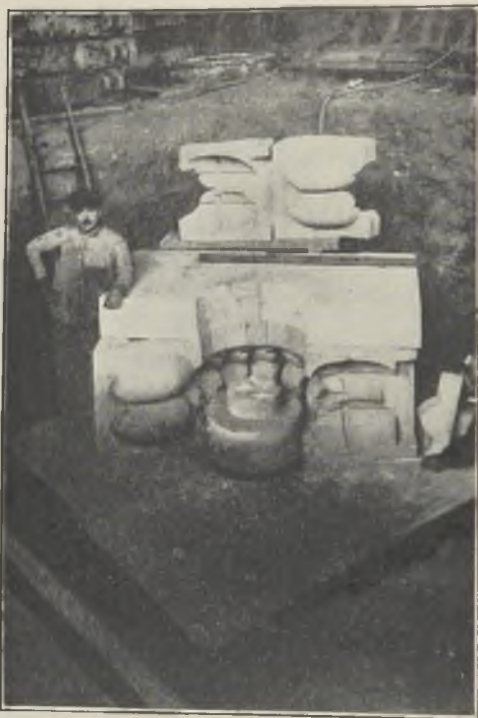
FIG. 20.—PUTTING TOGETHER PARTIALLY-STRUCK-UP RANDUPSON CASTING.
