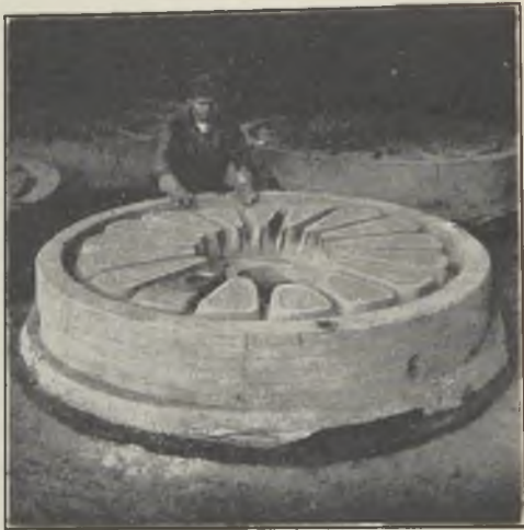
FIG. 28.—MOULD FOR LOCOMOTIVE WHEEL-CENTRE
