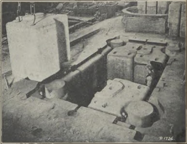
FIG. 11.—CORING-UP A "COMPO" MOULD FOR AN 80-TON STEEL PRESS CASTING.
