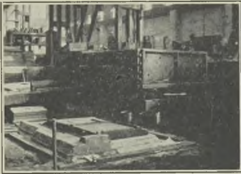
FIG. 14.—MOULD ASSEMBLY FOR GRINDING-MACHINE BED.
