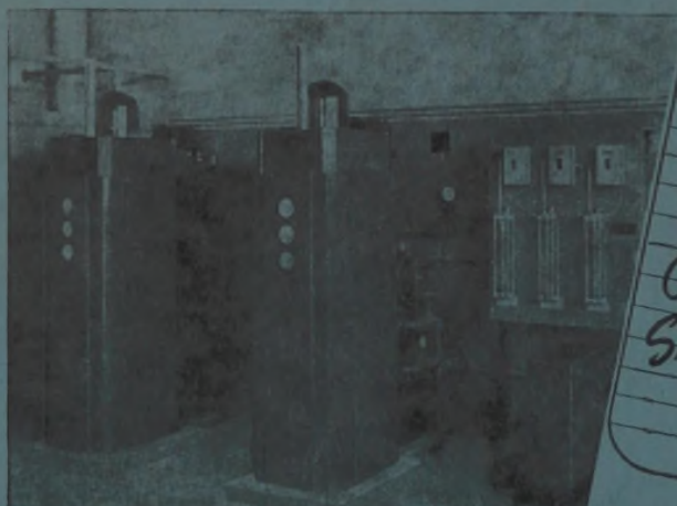
At Veterans' Home, Yountville, Calif., 2 Visible Vacuum Chlorinators prechlorinate on a schedule and chlorinate final effluent proportional to flow.
