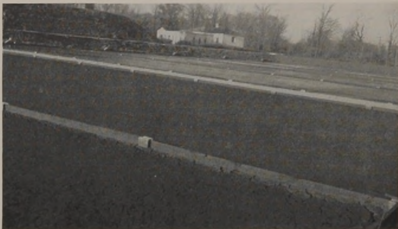
FIG. 3.—Shows the same sludge beds as in Fig. 2. Bed No. 7 left alum treated. Bed No. 6 at right no alum.
