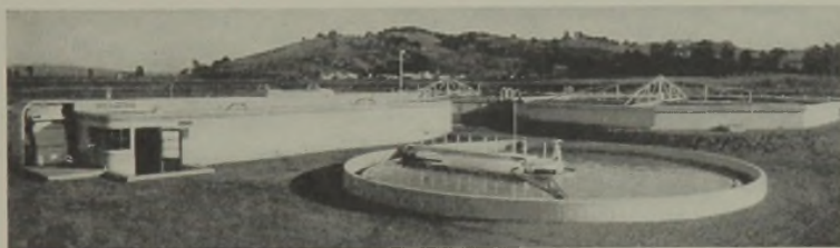
FIG. 1.—Dorr Biofiltration System at Petaluma, Calif. Primary Clarifier and Filter to right of building. Secondary to left and invisible.
