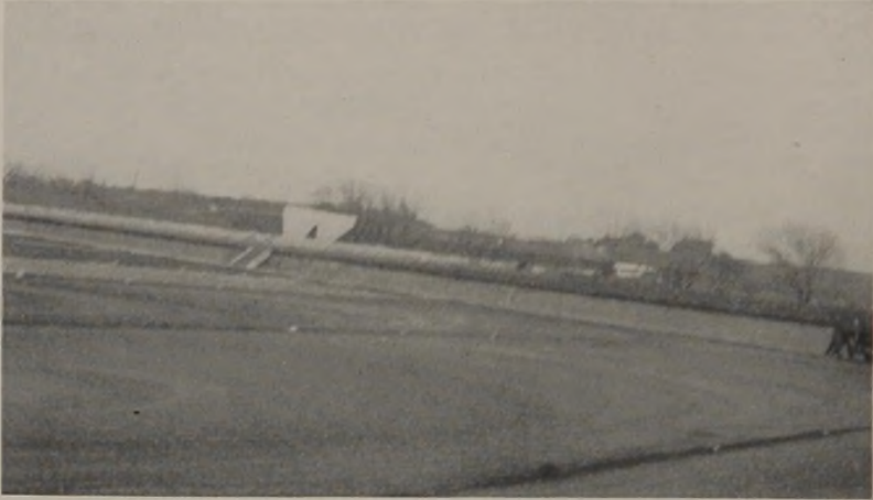
Fig. 1-A.—Appearance of alum treated sludge bed showing the typical “wrinkled” lumpy surface produced.
