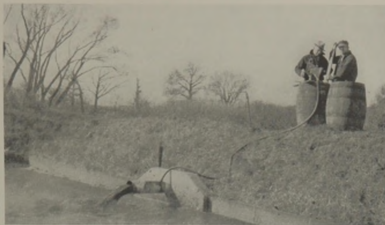
Fig. 6.—Shows the general method of applying alum to sludge beds as described in the text.
