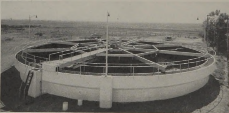
FIG. 2.—Dorreo Clariflocculator at Bakersfield, Calif.
