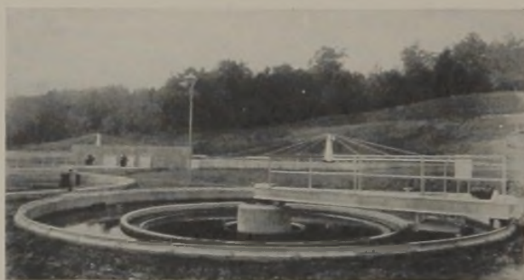
FIG. 3.—Liberty, N. Y. Downflow magnetite filter surrounding chlorination contact chamber for straining settled 2-stage bio-filtration effluent.
