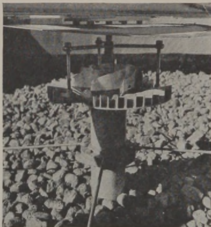
FIG. 2.—The Disc Distributor.
