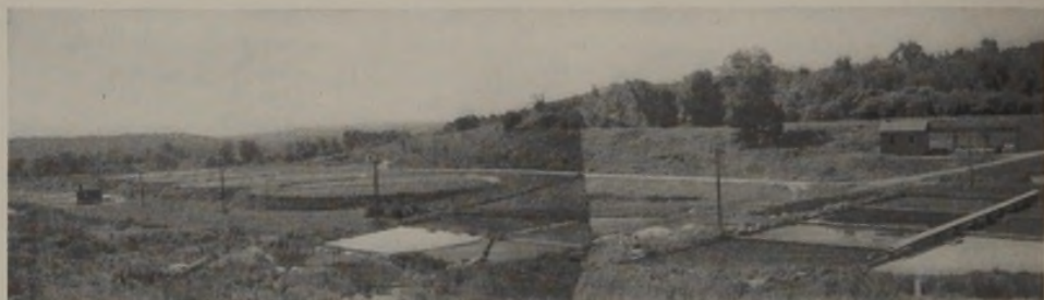
FIG. 1.—Sewage treatment works at Danbury, Connecticut, W. M. Kunsch, Superintendent.
