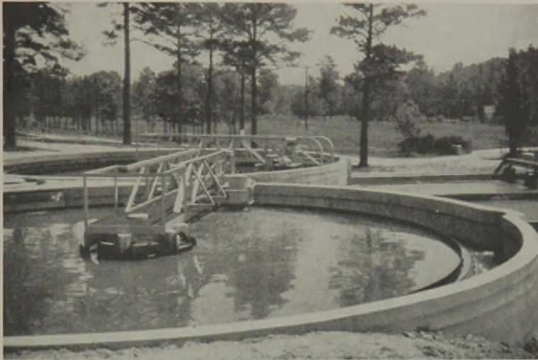
FIG. 2.—Two Primary PD Clarifiers at Fort McLellan, Anniston, Alabama.
