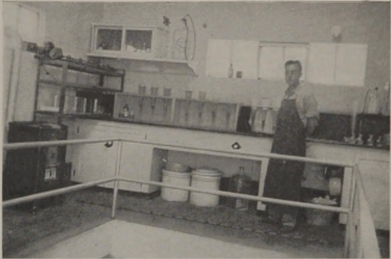
FIG. 9.—Laboratory. Palo Alto sewage treatment plant.
