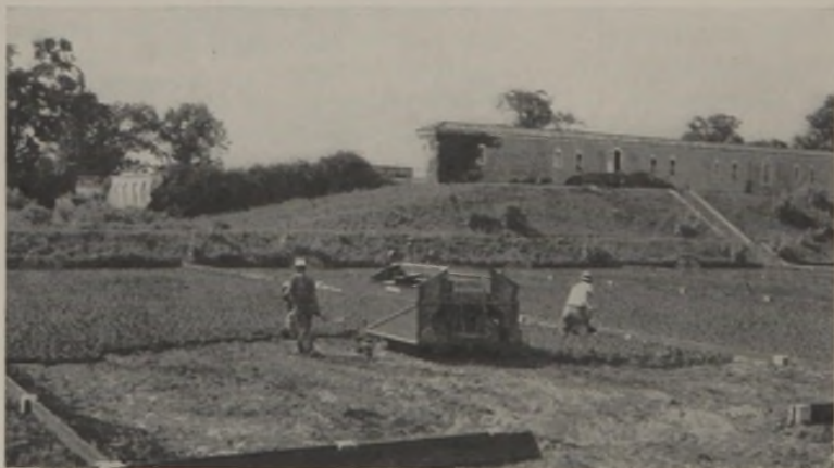
FIG. 3.—Aurora's Sludge Hauling Tractor in Service.
