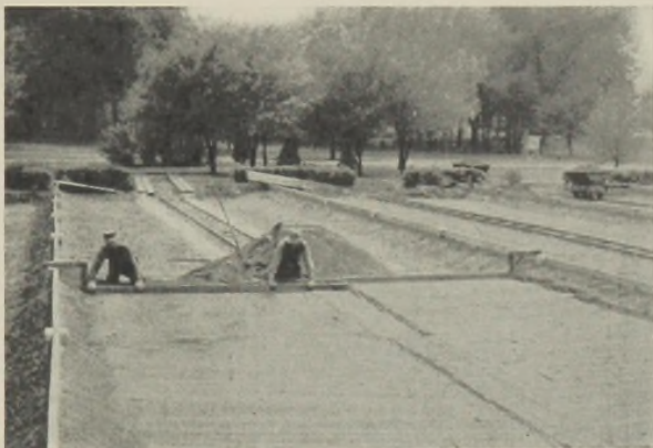
FIG. 4.—Resanding sludge drying beds.
