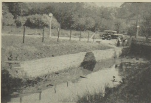
FIG. 2.—Retaining wall protecting section of sewer shown in Fig. 1.
