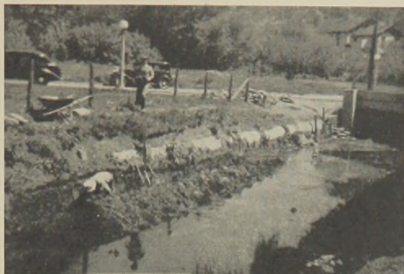
FIG. 1.—Intercepting sewer exposed by erosion.
