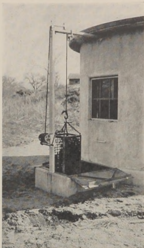
FIG. 1.—Basket screen hoisting assembly, Lisbon, South Dakota.
