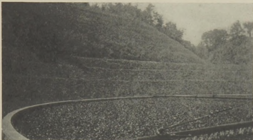
FIG. 4.—Sand bank shown in Fig. 3 after grading and seeding. Note terraces.
