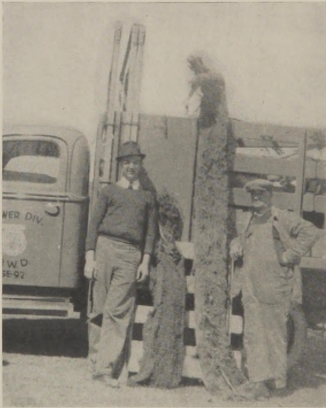
FIG. 2.—What sometimes clogs sewers.
