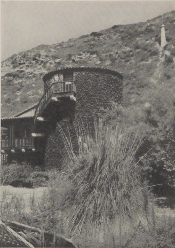
FIG. 3.—Same tower shown in Fig. 2 after planting with shrubs and vines.
