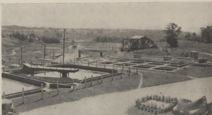
FIG. 1.—General view of plant. Foreground, left to right: Dorr settling tanks, Link-Belt settling tanks and digester, Dorr digester mound. Background: Trickling filters.
