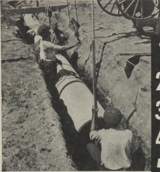
TRANSITE'S LONG LENGTHS facilitate laying pipe to accurate grades, speed up installation and reduce the number of joints in the line.
