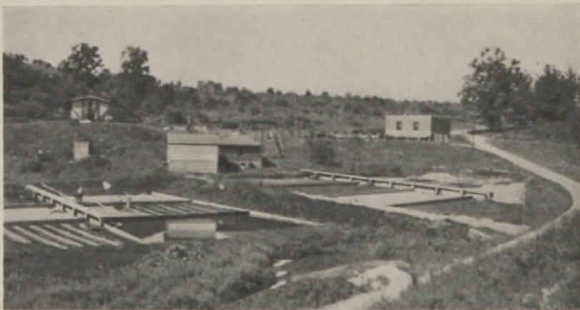
FIG. 2.—Foreground: Sludge drying beds. Background, left to right: Dorr digester mound, sludge control buildings, fine screen building.
