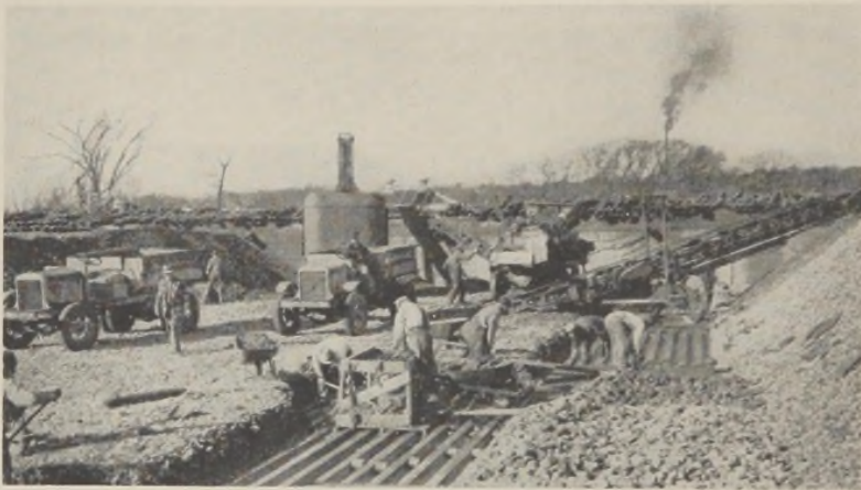
FIG. 3.—Hand screening of bottom layer of original stone.
