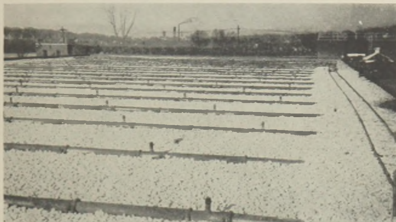
Fig. 4.—Restored filter prior to placing of granite surface layer.
