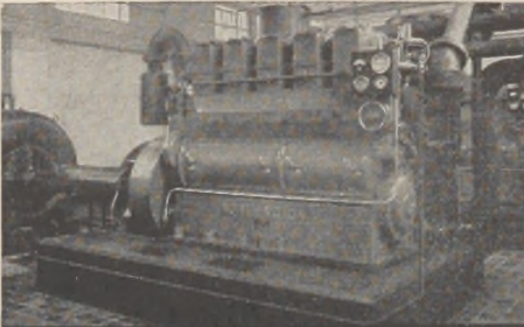
Sewage sludge gas engines
