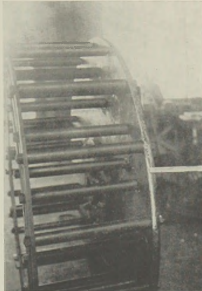
FIG. 2.—End view of cagemill showing joint between original and new plates.
