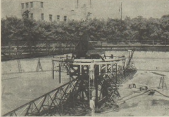
FIG. 6.—Installation of center wood baffle.
