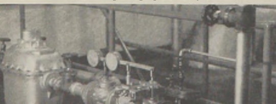
EMCO Meter measuring sewage gas used by boilers
