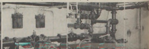
Nordstrom Valves on sludge lines in lower operating gallery between primary and secondary digestion tanks
