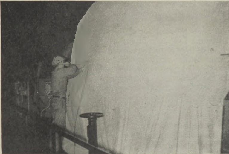
FIG. 3.—Placing sash cord segment insert during application of new cloth.
