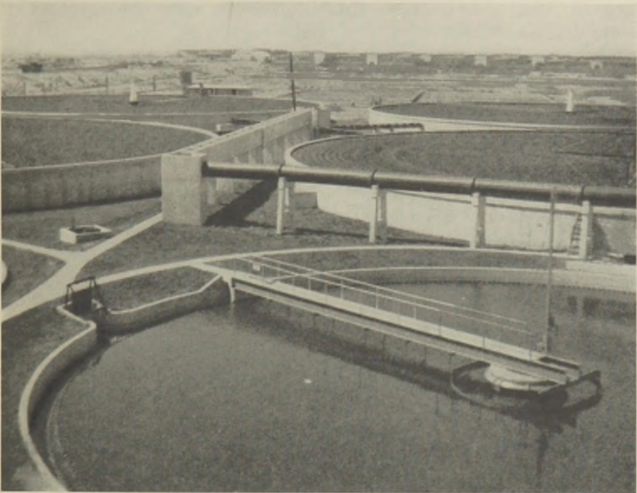
FIG. 1.—View of the trickling filters at Corpus Christi, Texas. One of the final clarifiers in foreground.
