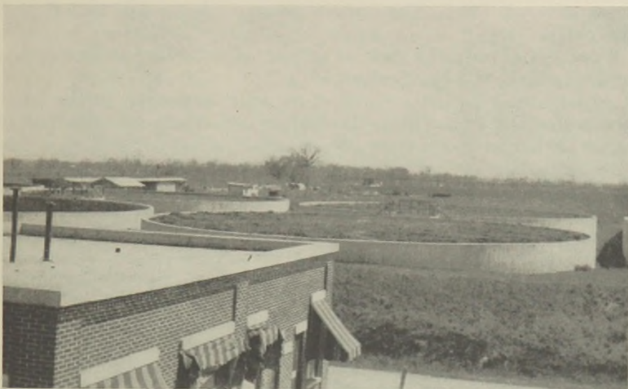
FIG. 1.—Four of the new open sludge digestion tanks at San Antonio, Texas.
