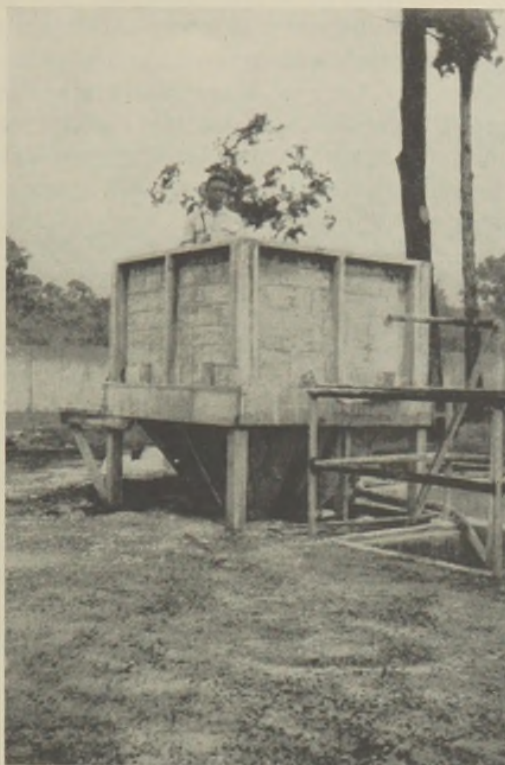
FIG. 2.—Chemical mixing hopper used in feeding chemical coagulants at an overloaded sedimentation tank.
