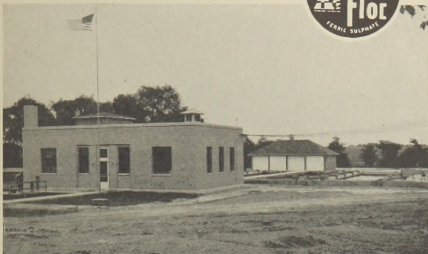
Elwood, Indiana, Sewage Treatment Plant
