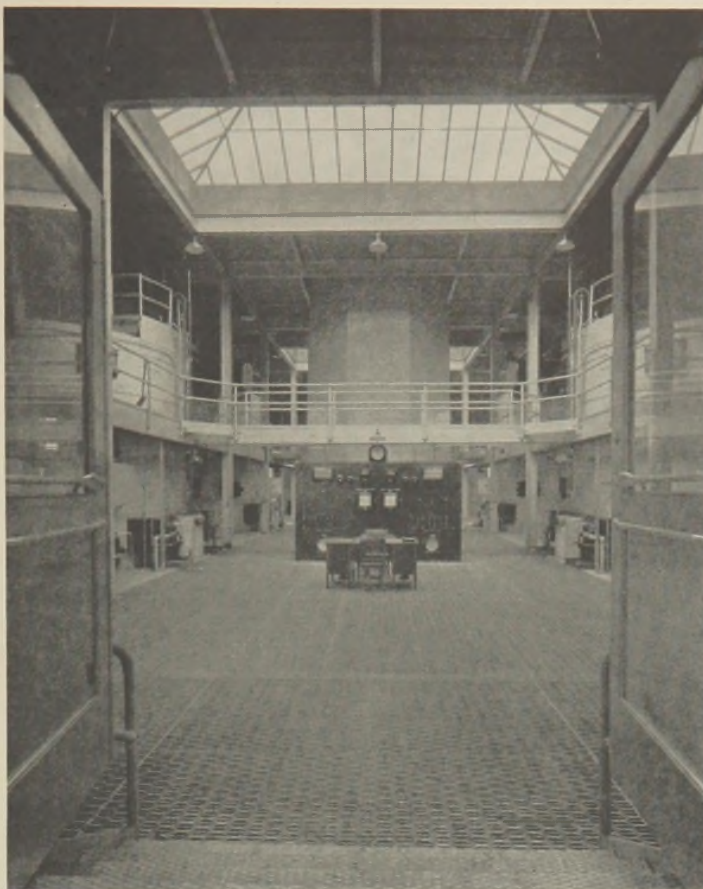
Fig. 3.—Aluminum floor grating, skylights, tread plate, conduit, and paint in Incinerator Building of Southerly Plant, Cleveland, O.
