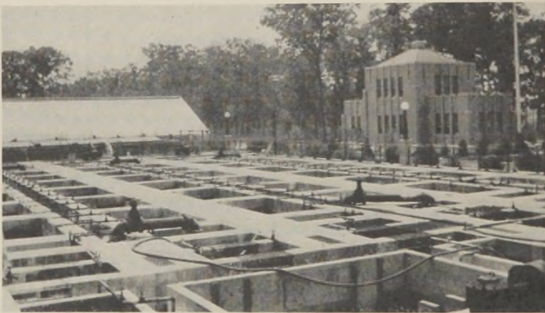
FIG. 1.—View of aeration tanks at Rockville Centre, N. Y. Blower house at right.
