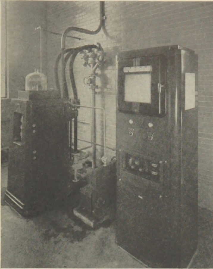
FIG. 1.—Wallace and Tiernan Potential Control Chlorinator Equipment at Fort Wayne, Ind., Sewage Treatment Works.
