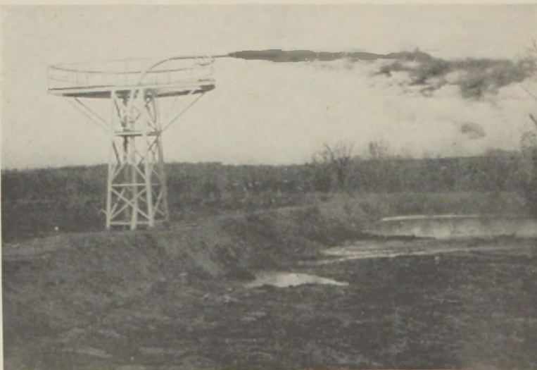
FIG. 3.—Pneumatic Ejector Discharge at South St. Paul.
