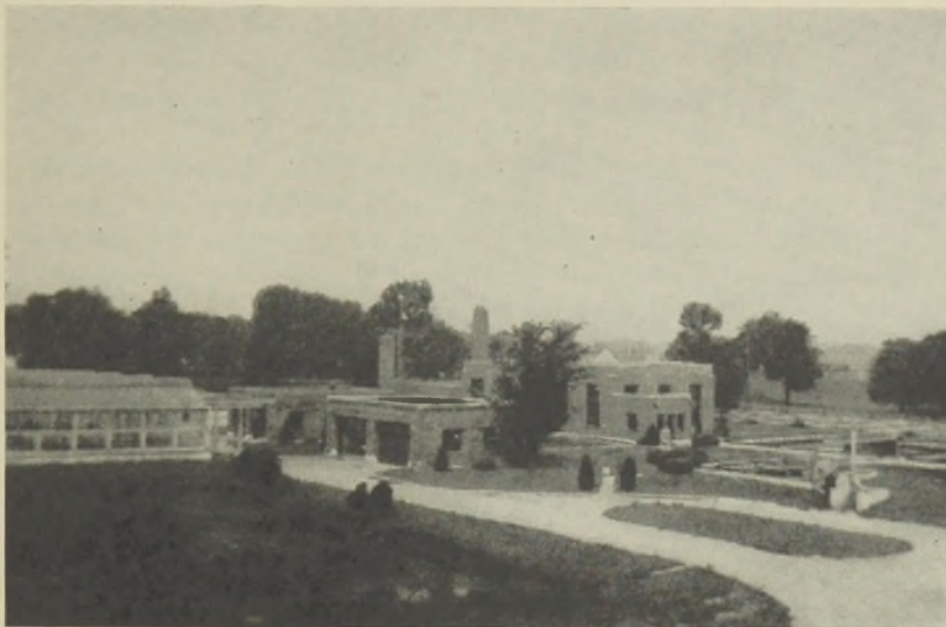
FIG. 2.—Findlay, Ohio aeration tanks at right rear, main building at center.
