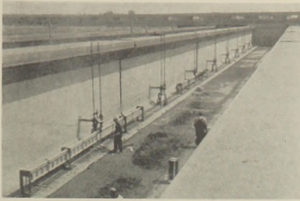
FIG. 3.—Installation of P.F.T. Aeration Plate Holder in Aeration Tank.
