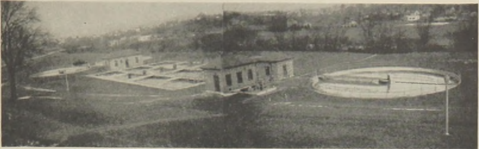
FIG. 2.—Sewage treatment works at Mansfield, Ohio. Primary settling tank at right.
