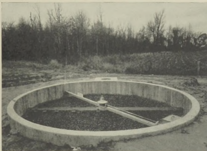
FIG. 1.—Yeomans Water-Wheel Distributor.
