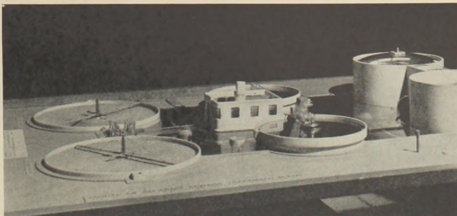
FIG. 1.—Two-Stage Biofilter Plant Model, built for the Corps of Engineers of the Army, Construction Division, Repairs and Utilities Branch.
