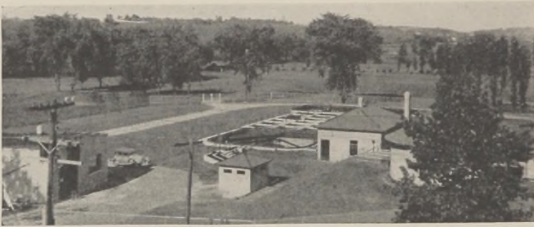
FIG. 1.—Activated Sludge Sewage Treatment Plant at Newark, N. Y. Designed by Glenn D. Holmes and Earl F. O'Brien, Syracuse, N. Y. Inertol Protective Coatings used on all concrete and steel structures.
