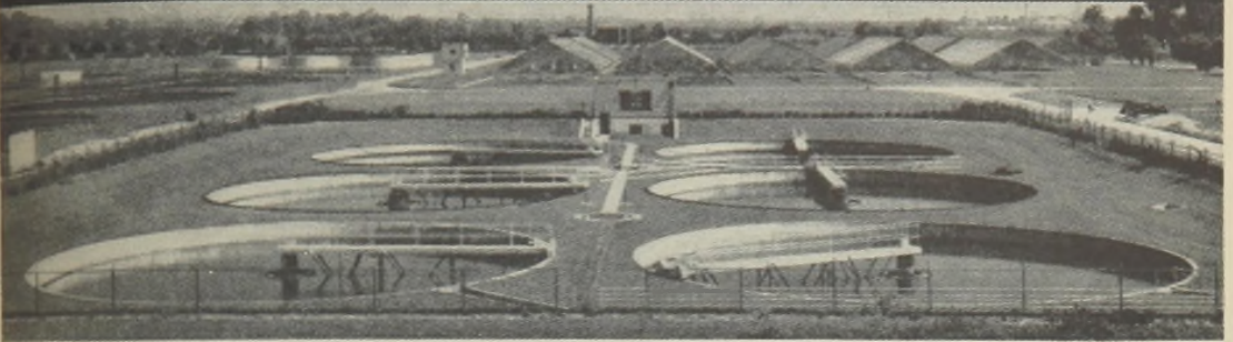
Dayton, Ohio sewage treatment plant showing six final tanks with Link-Belt Circuline Collectors in foreground.
