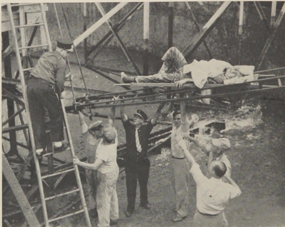
FIG. 1.—Proof that serious accidents do happen in sewage treatment plants.
