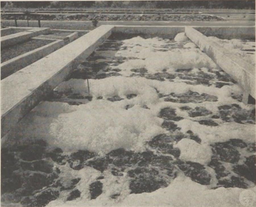
FIG. 3.—Surface of an aeration tank at an Army plant showing the distribution of air and the frequently characteristic foam.
