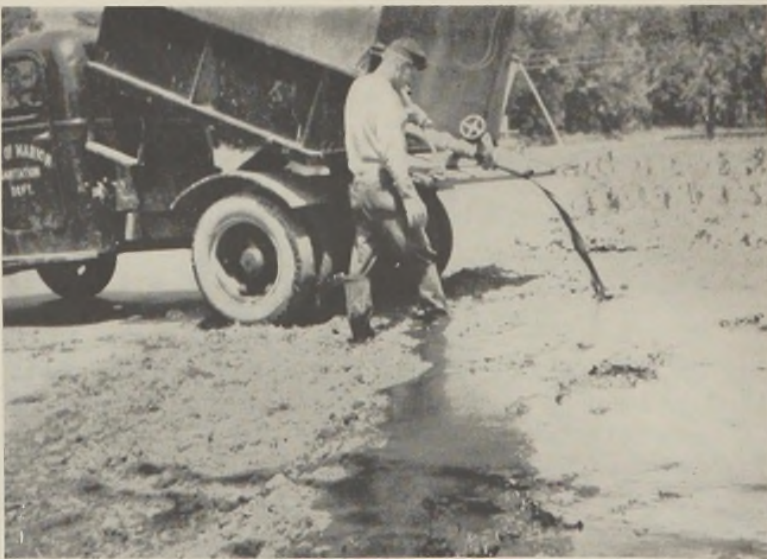
FIG. 2.—Marion, Indiana: Applying liquid sludge to farm land. Splatter plate attachment at end of drain pipe treats 6-foot strip when truck can be driven over area to be treated.
