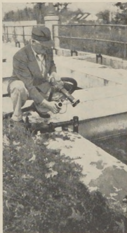
FIG. 1.—Arrangement for Flushing diffuser tubes with water at Rockville Centre, N. Y.
