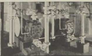
Vacuum pumps on sludge filters
