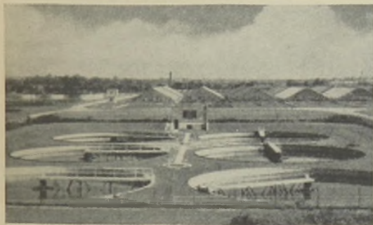
City of Dayton, Ohio sewage treatment plant. Showing six final tanks equipped with Link-Belt Circuline Sludge Collectors in this modern plant.
