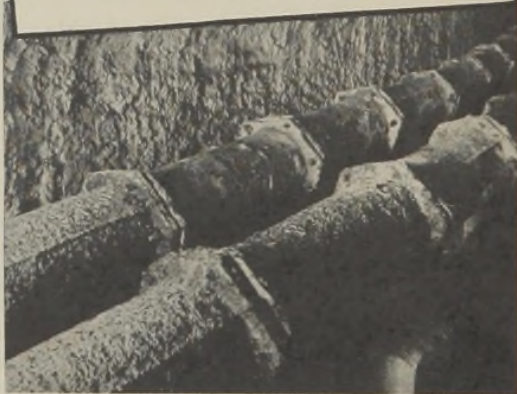
[Section of world's oldest cast iron water main still (at last reports) supplying the town and parks of Versailles, France, after 280 years of continuous service.]
