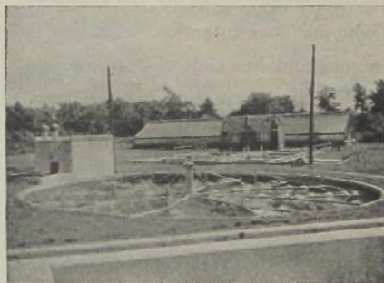
Rex Aero-Filter permits much larger daily capacities with smaller filter bed.
