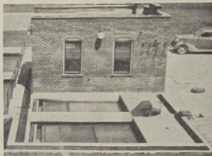
Small primary settling tanks equipped with Rex Conveyor Sludge Collectors.
