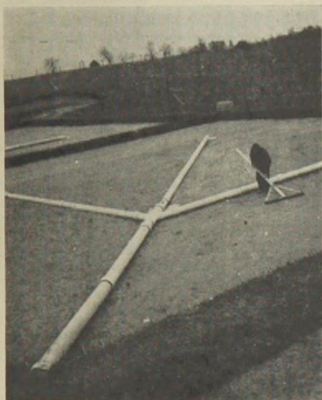
Class 50 Transite pressure pipe with Simplex couplings used as distribution piping for sewage filter beds in Ohio sewage treatment plant.
