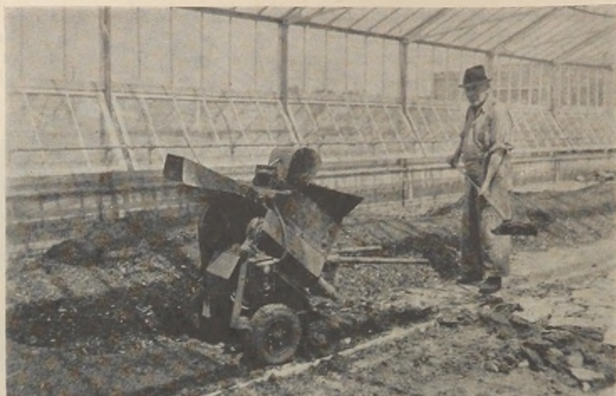
Fig. 2.—Converting sludge into fertilizer with a Royer at the Menominee, Michigan sewage treatment plant.
