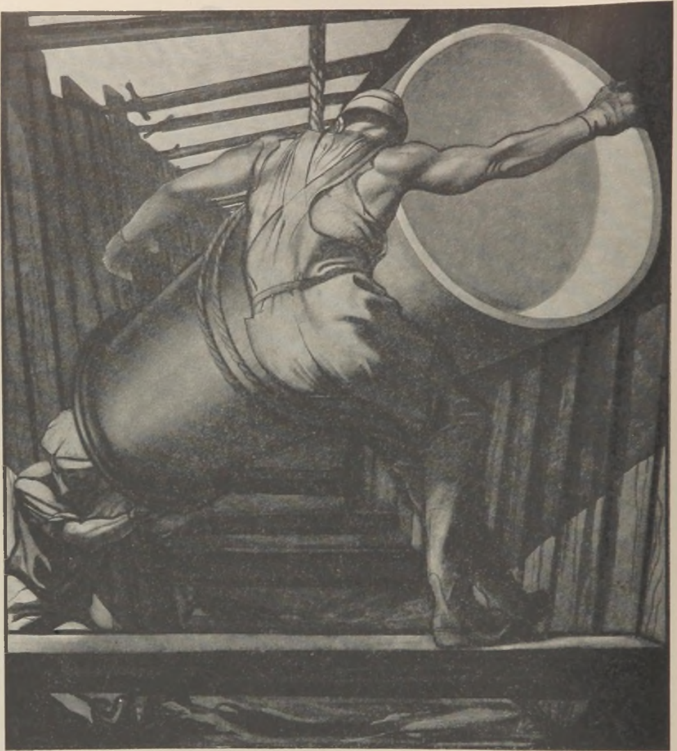
Installing cement-lined bell-and-spigot cast iron pipe. Drawn by Rico Lebrun for U. S. Pipe & Foundry Co.
