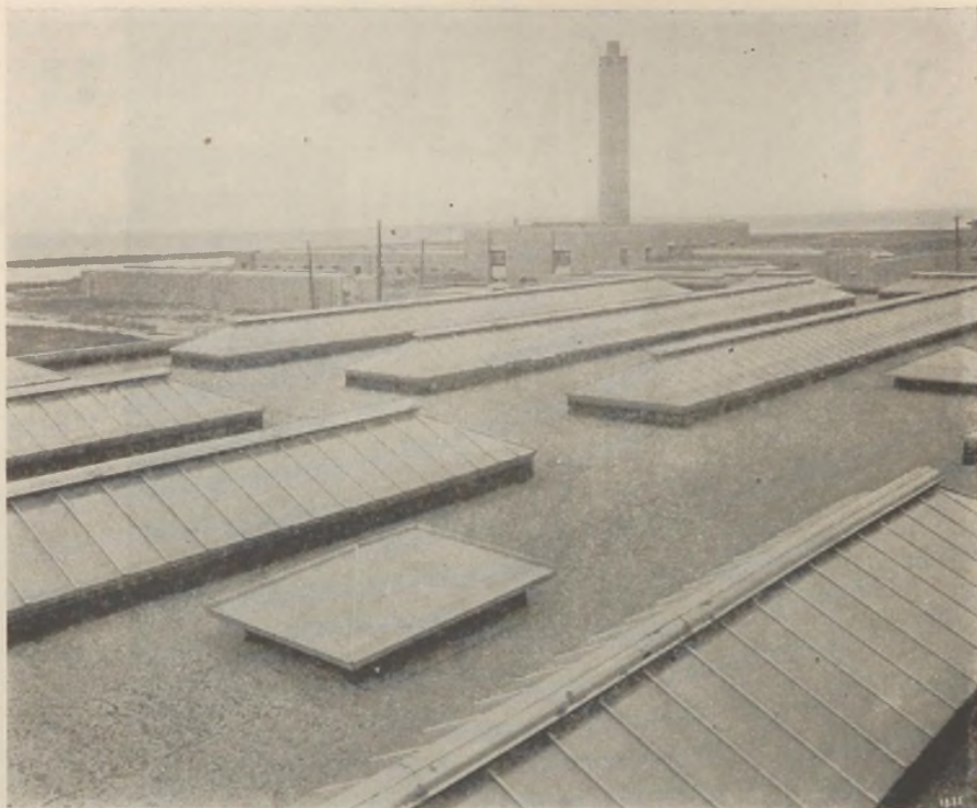
FIG. 2.—Aluminum skylights in use at Easterly Plant, Cleveland, Ohio. They are constructed entirely of extruded sections. The ridge member conceals a screened ventilating device operated from the interior.
