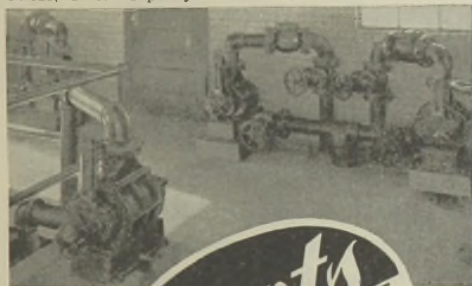
Four of eight "R-C" Meters for measuring sludge gas at Toledo, Ohio. Capacity of each 12,500 c.f. hr.
