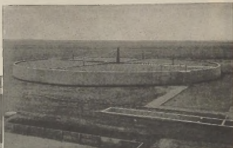
Above: 144 ft. diameter Graver Tricking Filter with Rotary Distributor.
