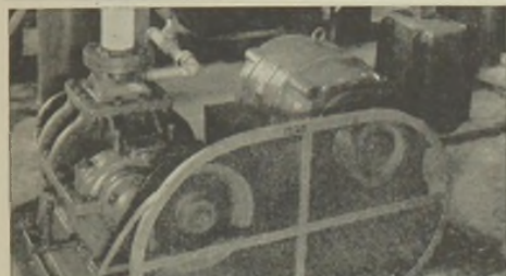
"R-C" Vacuum Pump installed at a New Jersey Sewage Treatment Works. Capacity 120 c.f.m., 20" mercury vacuum.
