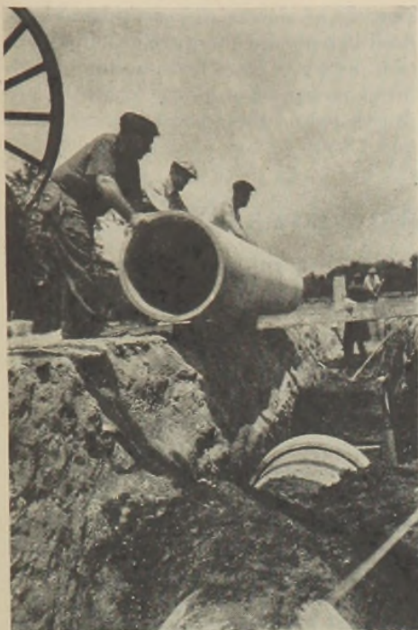
Long 13-ft. lengths of Transite sewer pipe are quickly and easily installed in Long Island. Tight, sleeve-type joints reduce infiltration to a minimum.
