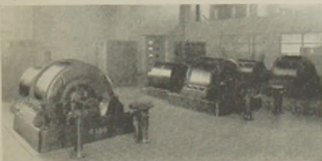
Three "R-C" Centrifugal Blowers driven by slip ring motors, installed at New York City. Capacity of each 15,000 c.f.m., 3,565 r.p.m., 7.75 lbs. pressure.
