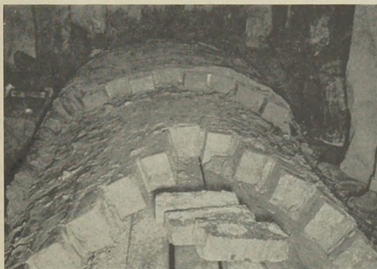
FIG. 2.—Repair of sewer arch illustrated in Fig. 1.
