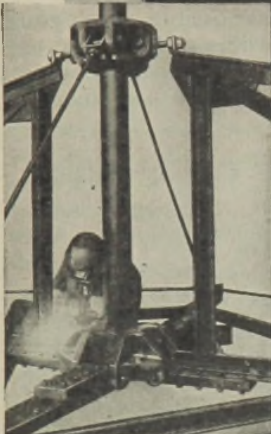
Fabrication of Sludge Scraper Mechanism
