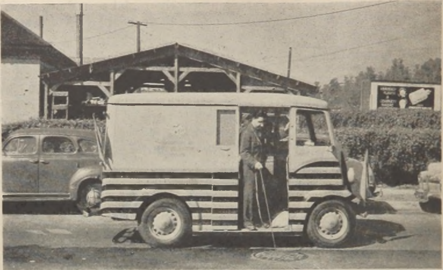
FIGURE 9.—Survey truck used for investigating explosive gas conditions.
