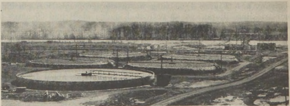
FIGURE 5.—Trickling filters and sedimentation unit treating phenolic wastes.
