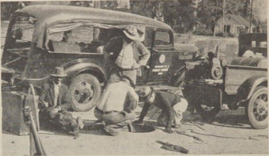
FIGURE 1.—Typical sewer maintenance truck used at Los Angeles.
