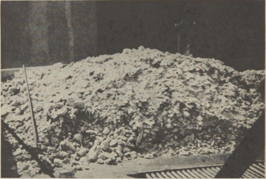
FIGURE 4.—Nine tons of grease removed from a 30-inch sewer in which a complete stoppage had occurred. Sold for $350 to the industry believed to have discharged it to the sewer originally.
