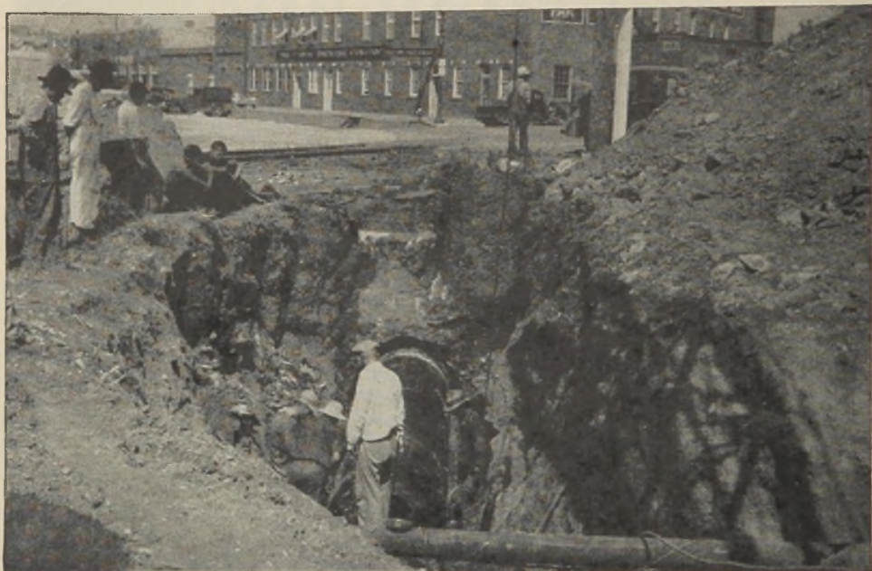
When the old sewer collapsed, a new trench was dug in 8 hours and in 10 more hours 188 feet of ARMCO Pipe was installed and backfilled. Long pipe lengths cut job time.
