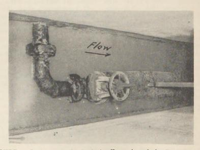
FIGURE 1.-Strainer at suction intake in effluent channel of sedimentation tank.
