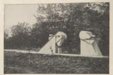
Rex "M.I." mechanically cleaned Bar Screen and Rex Grit Collector.
