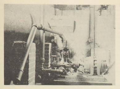
FIGURE 2.-Pump, pressure tank and piping used in effluent water system.
