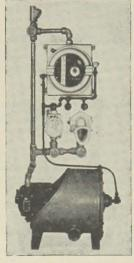
Alarm arranged for wall mounting. Instrument can be custom-built to meet special requirements.
