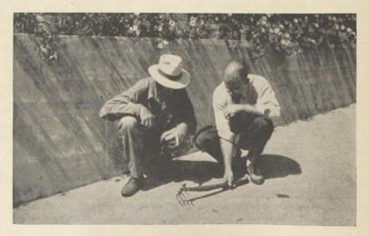
FIGURE 1 .- "Rag Picker" gadget for removing accumulations from clarifier weirs.
