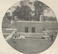
Small primary settling tanks equipped with Rex "M.I." Conveyor Sludge Collectors.
