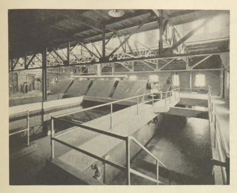
FIGURE 10 .--- View of grit chambers at Racine, Wis. Washer at right.
