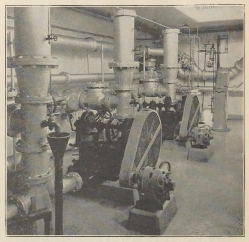
Showing CLOW CAST IRON flanged pipe and fittings installed in the Sewage Treatment Works for the City of Grand Rapids, Michigan.
