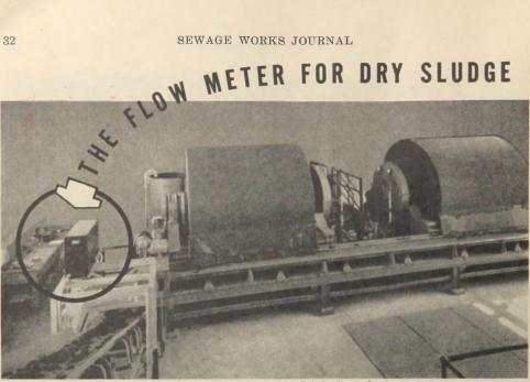
Toledo-Chronofio Conveyor Scale weighing sludge cake at Cranston, R. I. Sewage Treatment Works. Photo courtesy EIMCO CORP.
