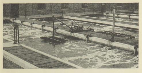
Chicago Wide Band Air Diffusion System with Swing Diffusers at Omaha, Neb., Sewage treatment plant.
