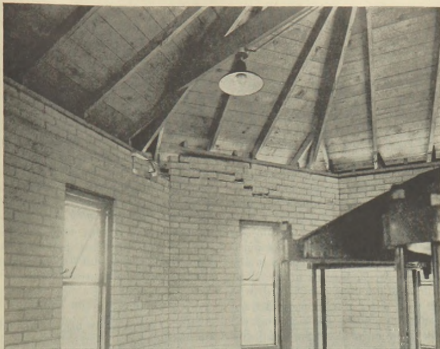
FIGURE 2.—Interior of building damaged by digester gas explosion at Traverse City, Mich.
