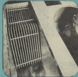
Aluminum's resistance to corrosion recommends its use for bar screens.
