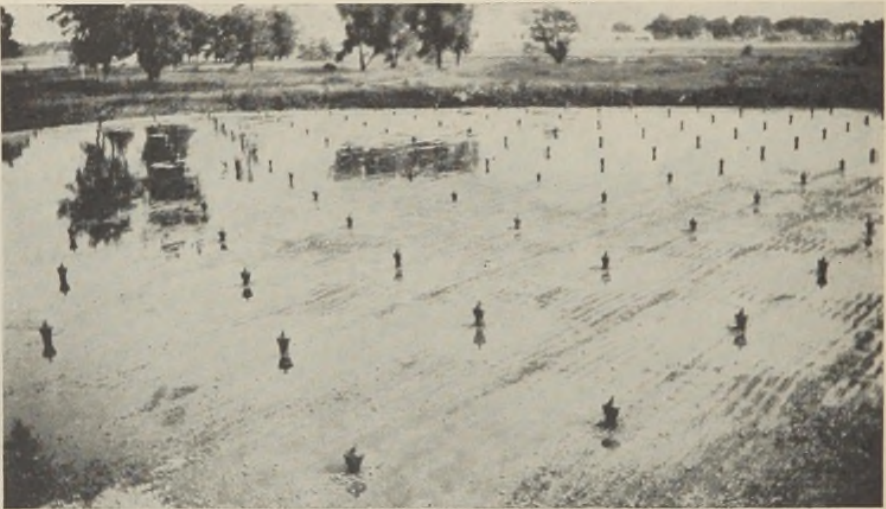
FIGURE 2.—Badly pond trickling filter at Madison, Wis. Fine surface media and overloading by packinghouse wastes responsible.
