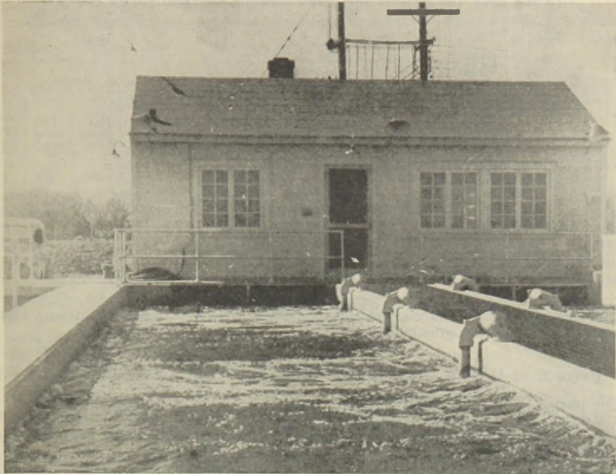
PLATE 21.—Aeration basins in activated sludge plant at Lake Charles AAF, La.
