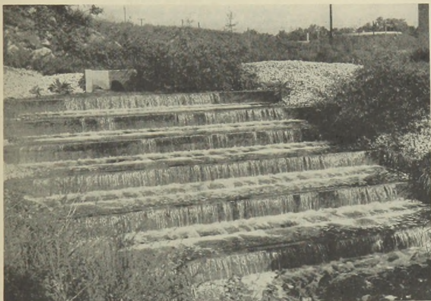
PLATE 16.—Aeration ladder for plant effluent, Fort Knox, Ky.
