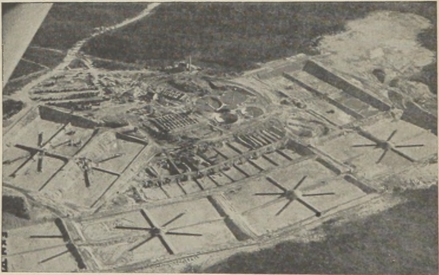
FIGURE 5.—Large trickling filter plant, Camp Edwards, Mass. Units in foreground are sand beds that completely absorb effluent into ground.
