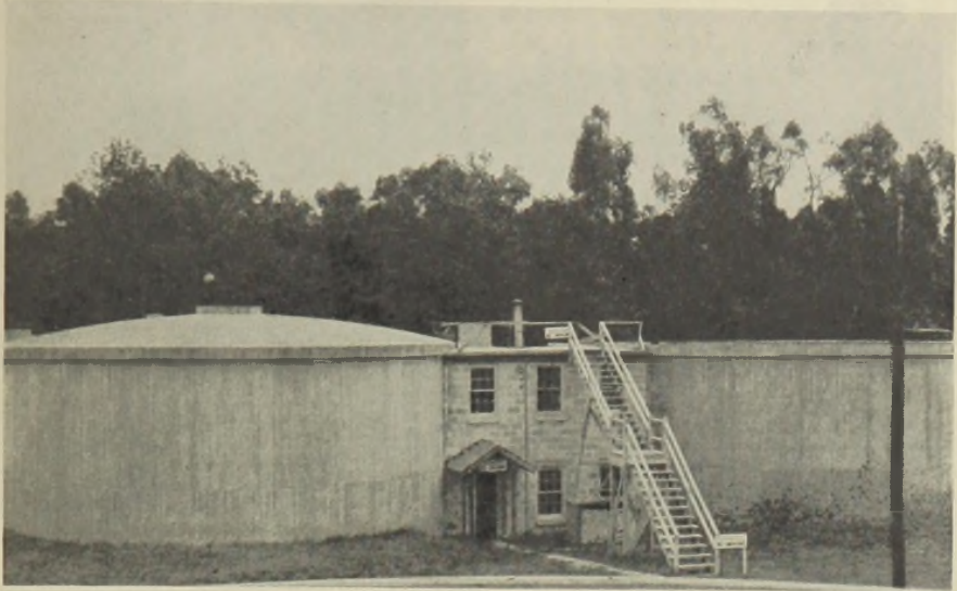
PLATE 23.—Sludge digesters at Camp Plauche, NOPOE, La.
