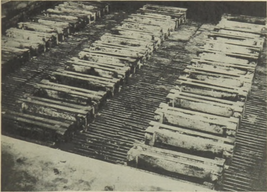
PLATE 18.—Contact aerators, showing plate arrangement at Hondo AAF, Texas.
