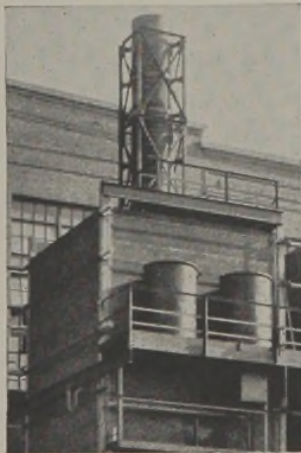
47' high all-carbon electrostatic precipitator
